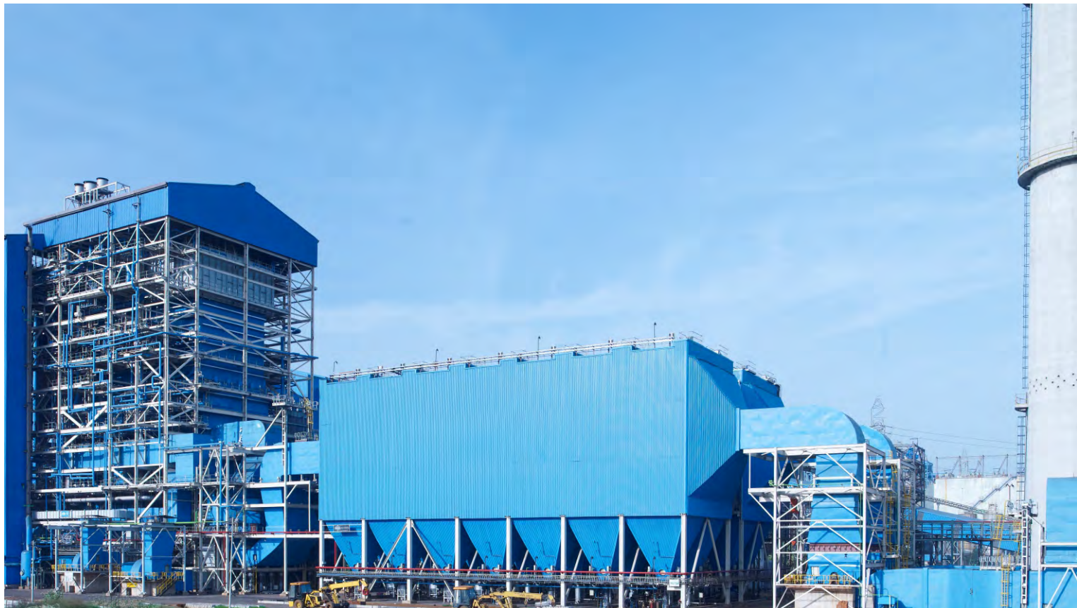
180 Mwe Pulverized Coal Fired Boiler with Reheat firing 100% Indonesian Coal & 100 % Indian Coal for OPG Power Generation Pvt. Ltd., Chennai, India
