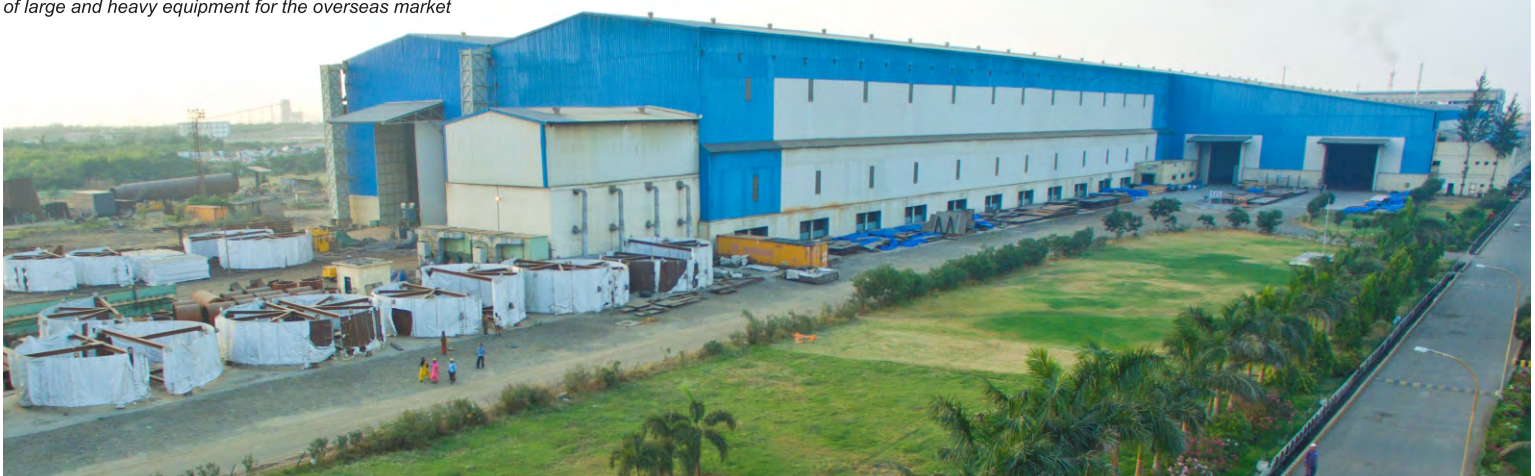
Isgec Plant at the port town of Dahej (Gujarat) India. The shop has been set up especially for the manufacture of large and heavy equipment for the overseas market
