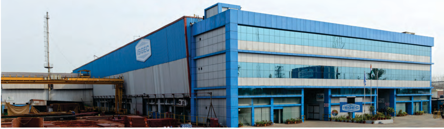
Boiler Pressure Parts Plant at Rattangarh (Haryana) India The Plant has a covered Shop Area of 16,650 sq.m. We also have additional adjoining land area for quick & easy expansion
