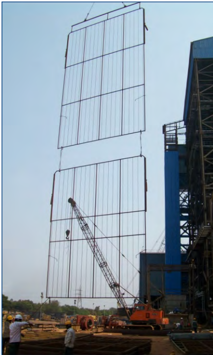
Discharge Frame with VARIODYN 15 Electrodes
