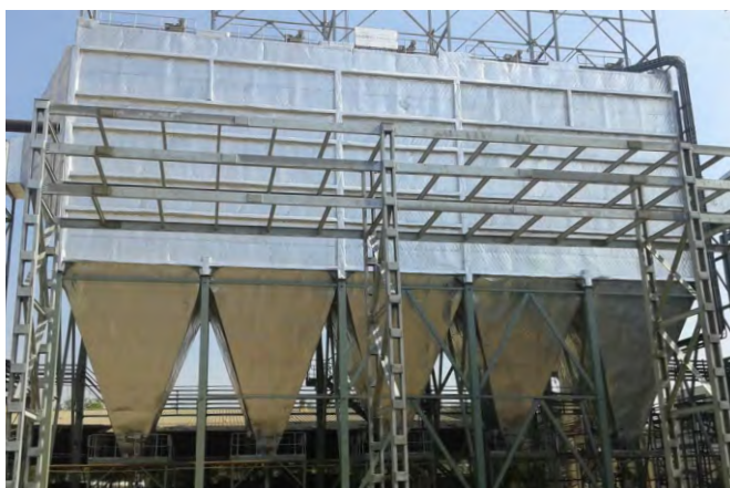
35 MW CFBC Power Plant at United Phosphorus Ltd., Gujarat
