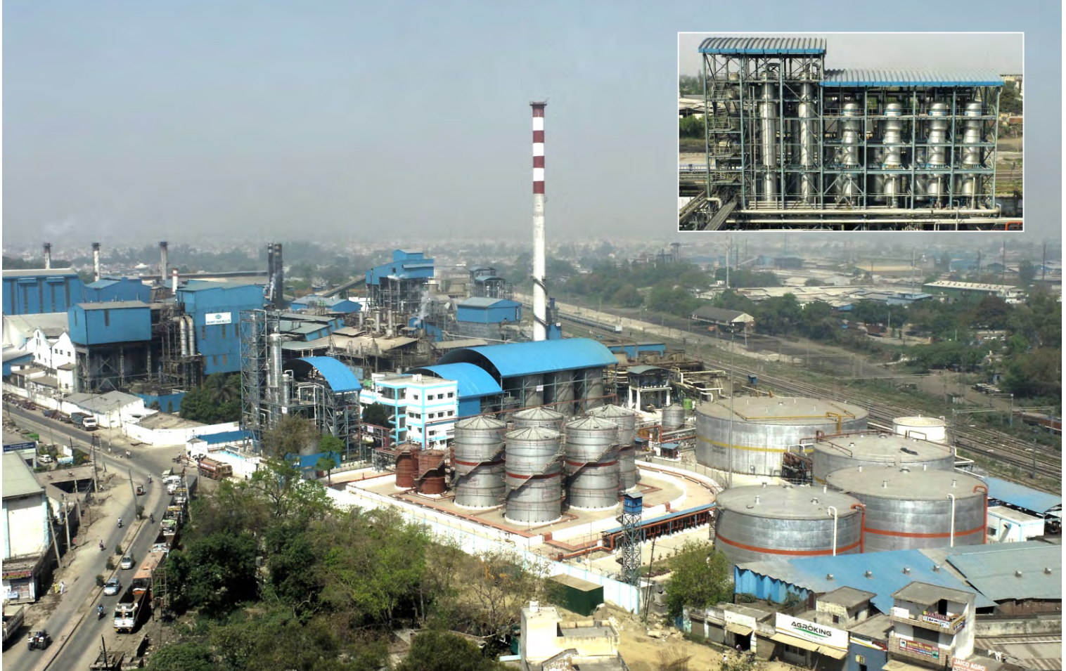
160 KLPD Multi-Feed Distillery with 48 TPH Slop Fired Incineration Boiler and 5.6 MW Power Plant on complete EPC basis including Civil Work at Saraswati Sugar Mills Ltd., (Haryana), India
