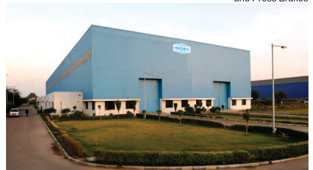
Plant at Bawal (Haryana) India for manufacturing Standard GAP Frame, H-Frame Mechanical Presses and Press Brakes
