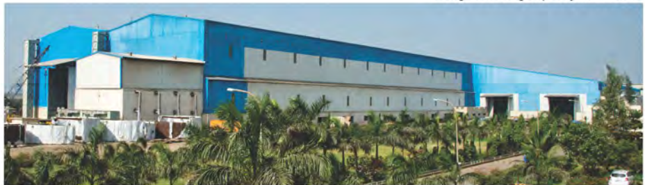
Coastal facility at the port town of Dahej (Gujarat) India with a lifting / handling capacity of 300 MT.
