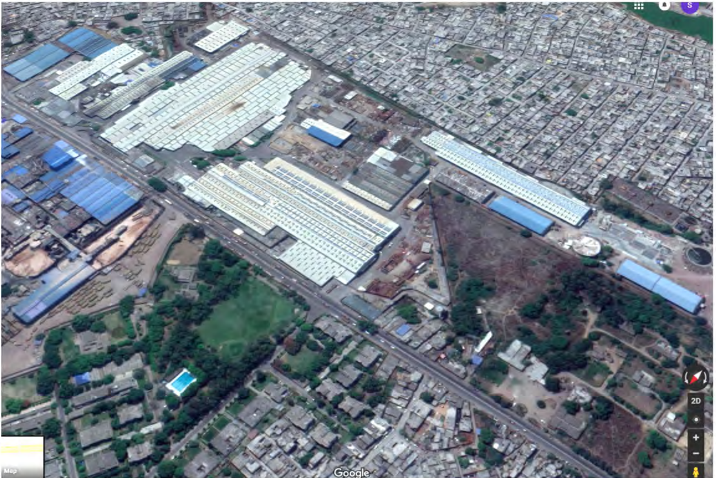
A Google Earth view of the Isgec Plant at Yamunanagar (Haryana) India.
