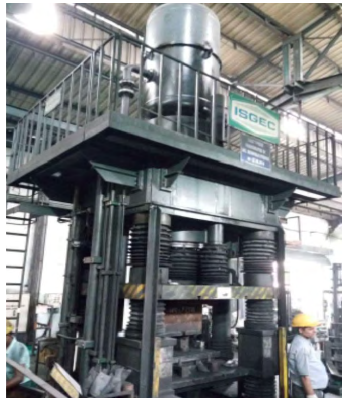
2000T Press for Refractory Bricks, Nozzles & Slide Gate Manufacturing
